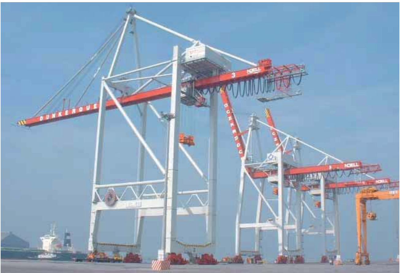
VAHLE Motor Reelers and Festoon Systems, container cranes at Dunkirchen Harbour
