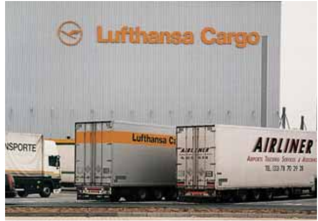
Airport Cargo Terminal
