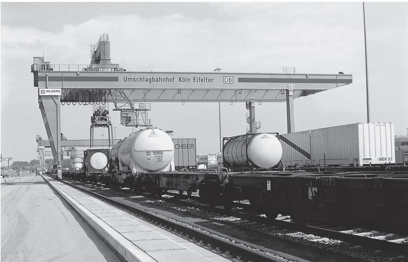
VAHLE-EID conductor trench for container terminal
