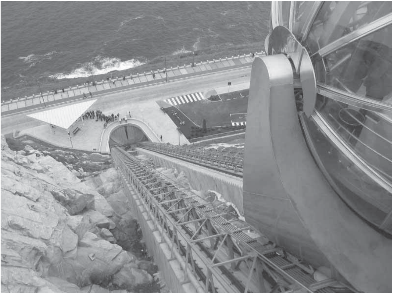
Inclined elevator A Coruña
